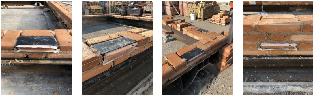
Figure 5.1: Illustrations of the deployment of smart bricks of standard dimensions.
