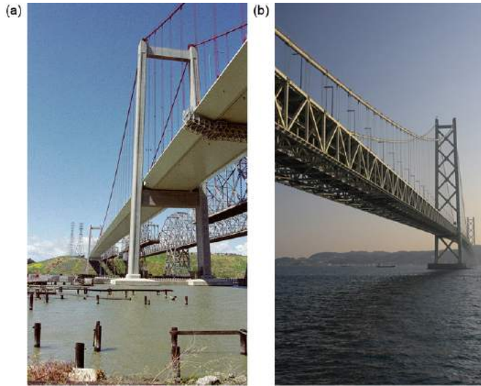
Figure 4.6: Photo of the New Carquinez Bridge (a) and of the Akashi Kaikyo Bridge (b).
