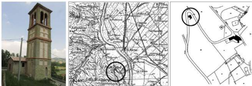
Figure 3.6: View of the bell tower of the Ponte Pattoli's "Old" church and cadastral maps maps (Ponte Pattoli, Perugia, Italy).
